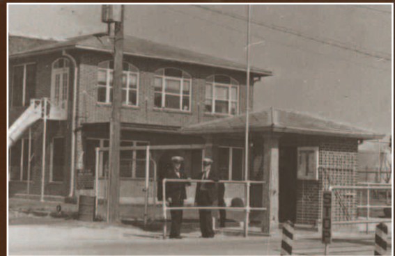
The Main Office Building and early security gate were constructed in 1920 and served the Refinery until 1964.
