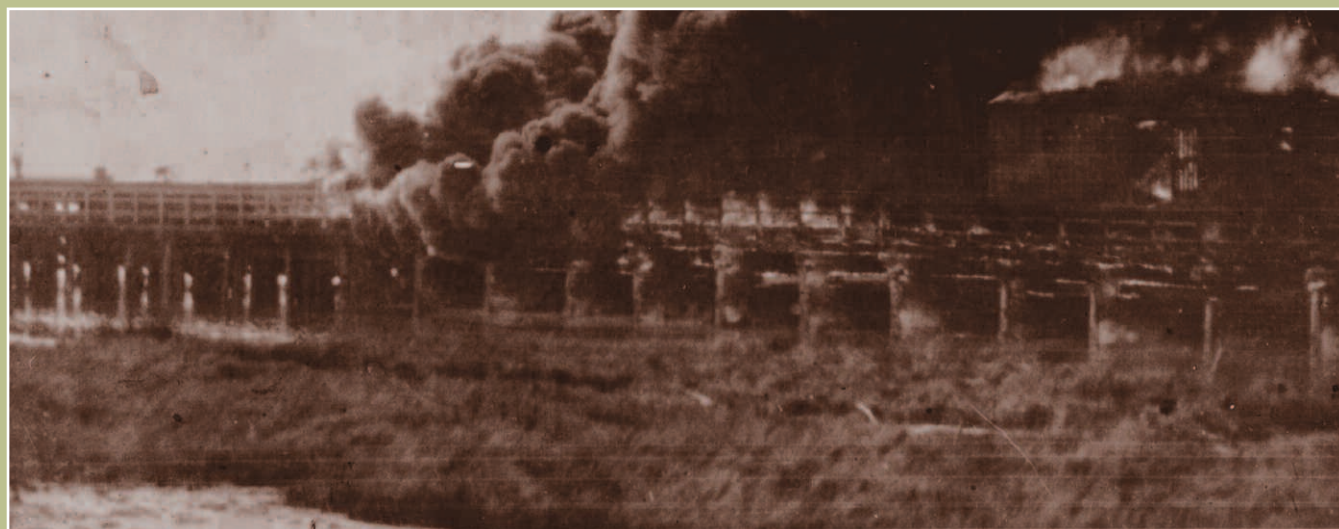
The no. 1 wooden dock burned in 1920 and was replaced with concrete.
