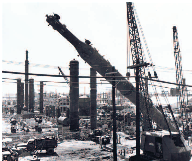
Another tower is raised at CLEUs-3 in 1957 to add to the forest of towers in that area.
