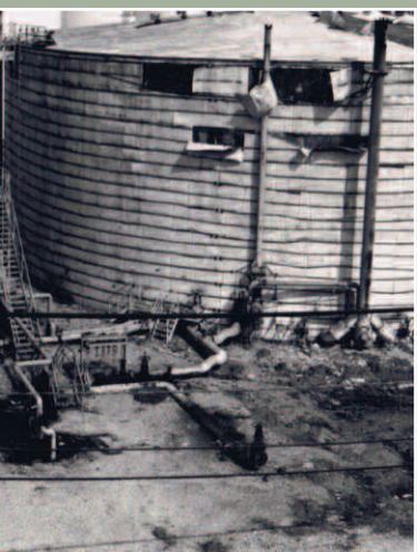
In August 1983, Hurricane Alicia struck the Complex with Category 3-force winds, causing an extensive amount of damage.
