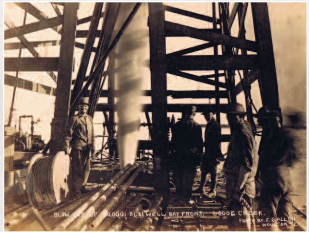
Blow-out of a 30,000 barrel well at Goose Creek Oil Field. First came natural gas or salt water under great pressure, followed by a fountain of oil. This well could possibly be the famous sweet No. 11.
