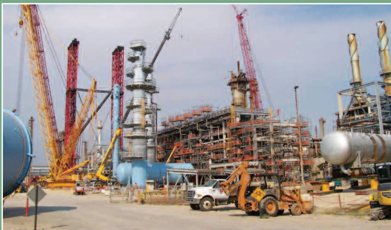
Construction on Hydrofining Unit 10
