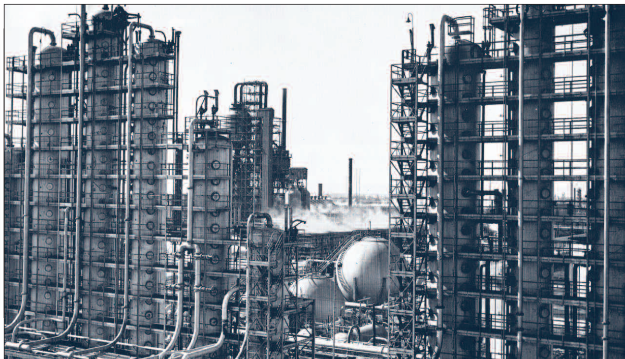
In this wartime view of the Refinery in the 1940s, the light-ends fractionating towers are seen in the foreground and the toluene facilities at BOW in the background.
