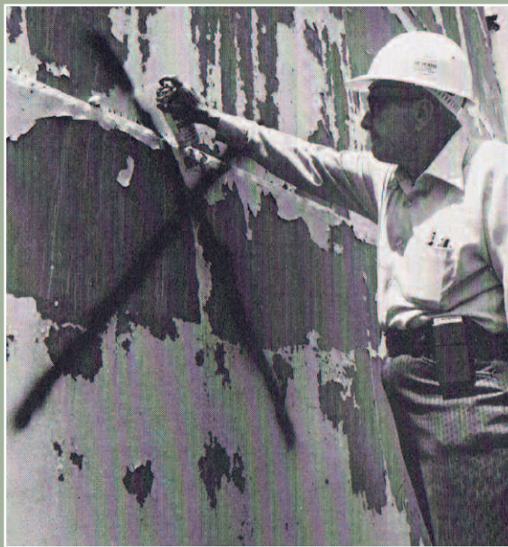
Oil Movements Chief Operator L.H. Hales applies a big "X" on a tank, which meant it would be torn down as part of a storage tank modernization program to replace 100 tanks with 36 larger tanks by 1975.
