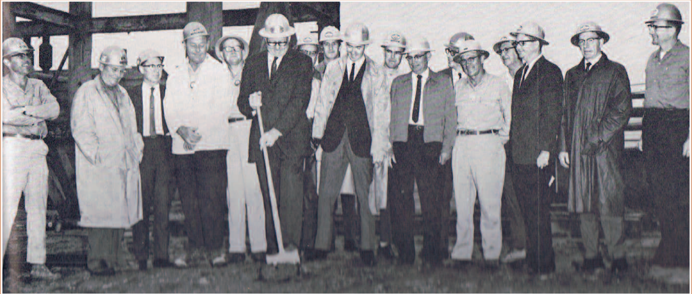
In 1965, a groundbreaking ceremony was held for the new hydrocracking unit. Pictured are, left to right, J.H. Dunn, Rigging; E.T. Davis, M&C; Frank Darrow, contractor rep; Pete Hargrave, M&C; E.E. Buchschacher, FCCU-3; H.H. Meier, refinery manager; C.J.H. Wahlstrom, Technical; H.M. Arno, Technical; G.P. Reynolds, Fuels; W.B. Nethery Jr., Technical; B.S. Greenwood, Fuels; E.L. McGee, Technical; L.D. Meckel, FCCU-3; John Moore, Technical; R.P. Larkins, Fuels; A.B. O'Brien, Purchasing; L.D. Braswell, Technical.
