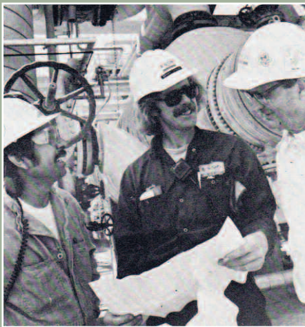
Process employees Willie Olivarez, Gerry Miller and Andy Page begin start-up of the BTFE equipment at crude light-ends facilities.
