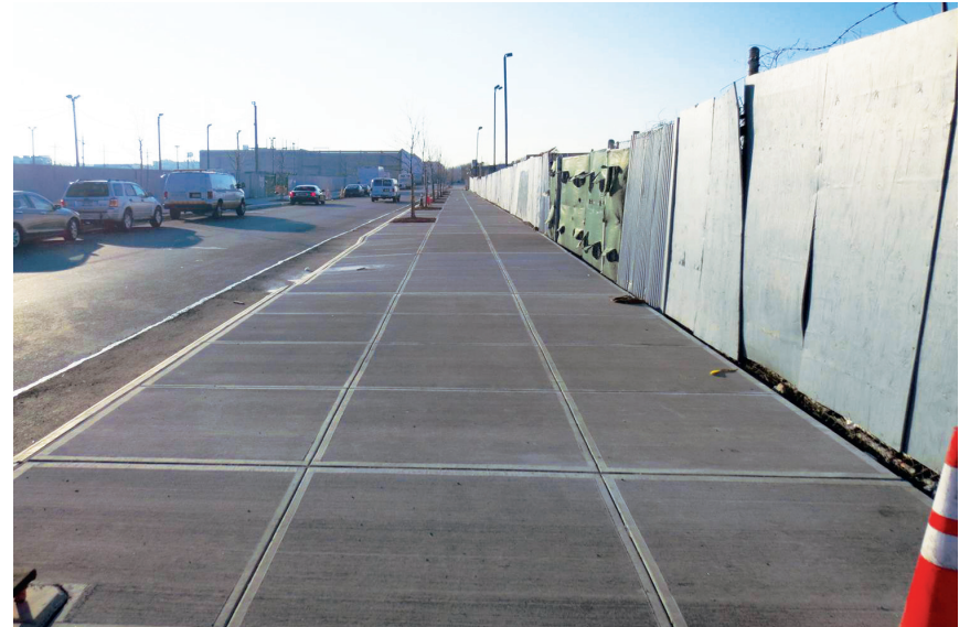
A view down the new Monitor Street sidewalk
