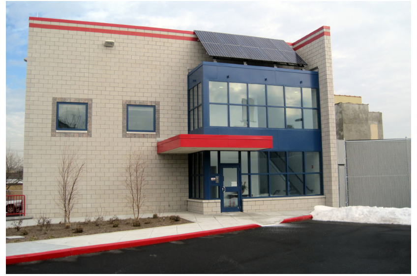
Solar Panels on SVE building ExxonMobil uses solar panels on its new Soil Vapor Extraction facility to produce 30,000 watts of energy, enough to supply the needs of the facility's office space.
