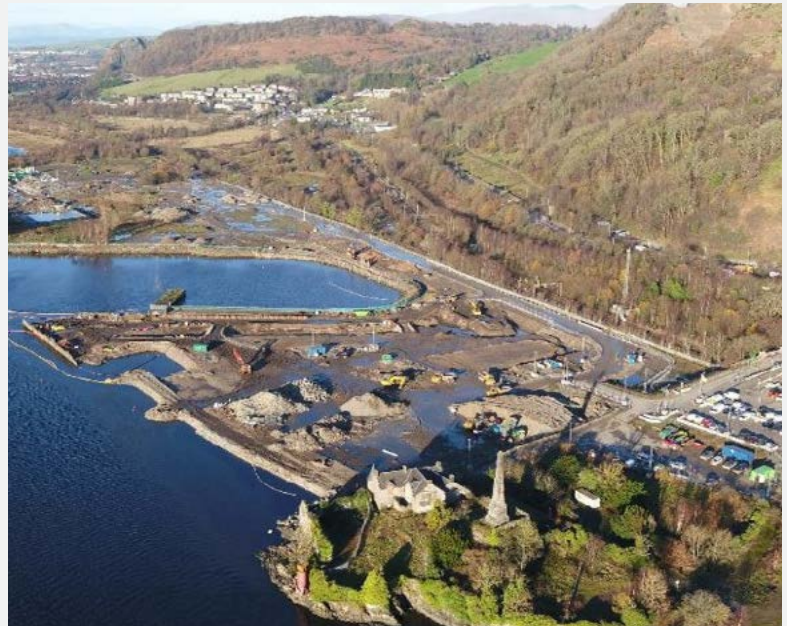
Photo: Aerial view of Bowling remediation site.
