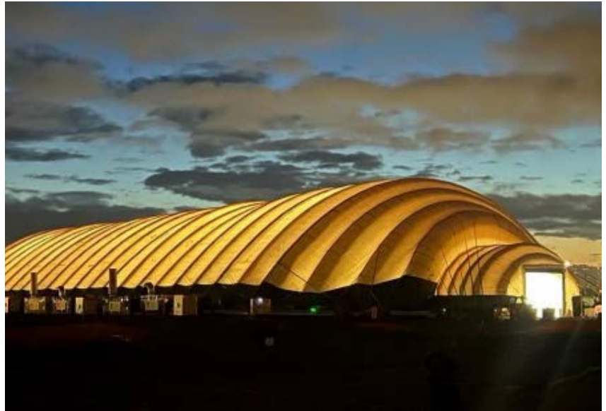
Photo: Inflatable tent deployed in France when decommissioning a World War II-era refinery.
