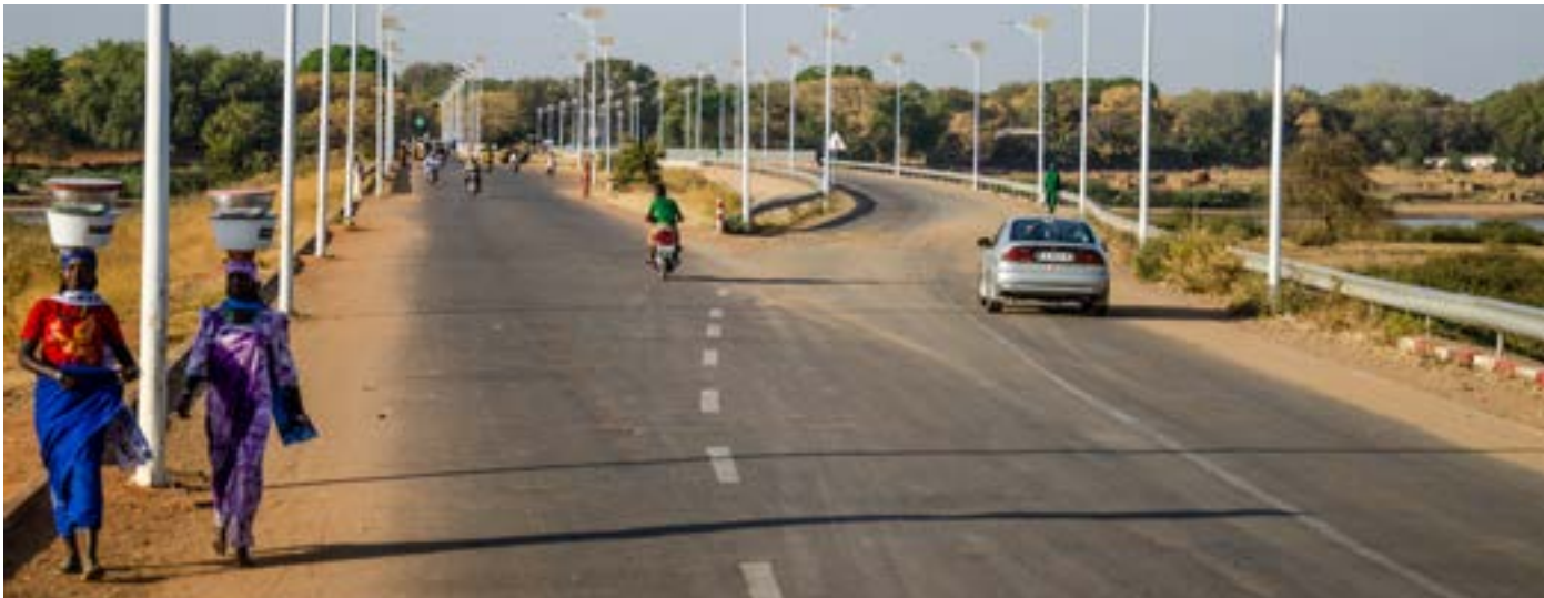
The recently completed Moundou Bridge allows traffic to flow to and from the city simultaneously, removing an important bottleneck to commercial activity in the city. Oil revenues were the source of the 10.2 billion FCFA the Chadian government invested in building this 370-meter-long bridge.
