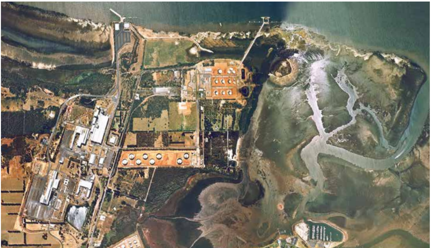
Long Island Point plant from above.
