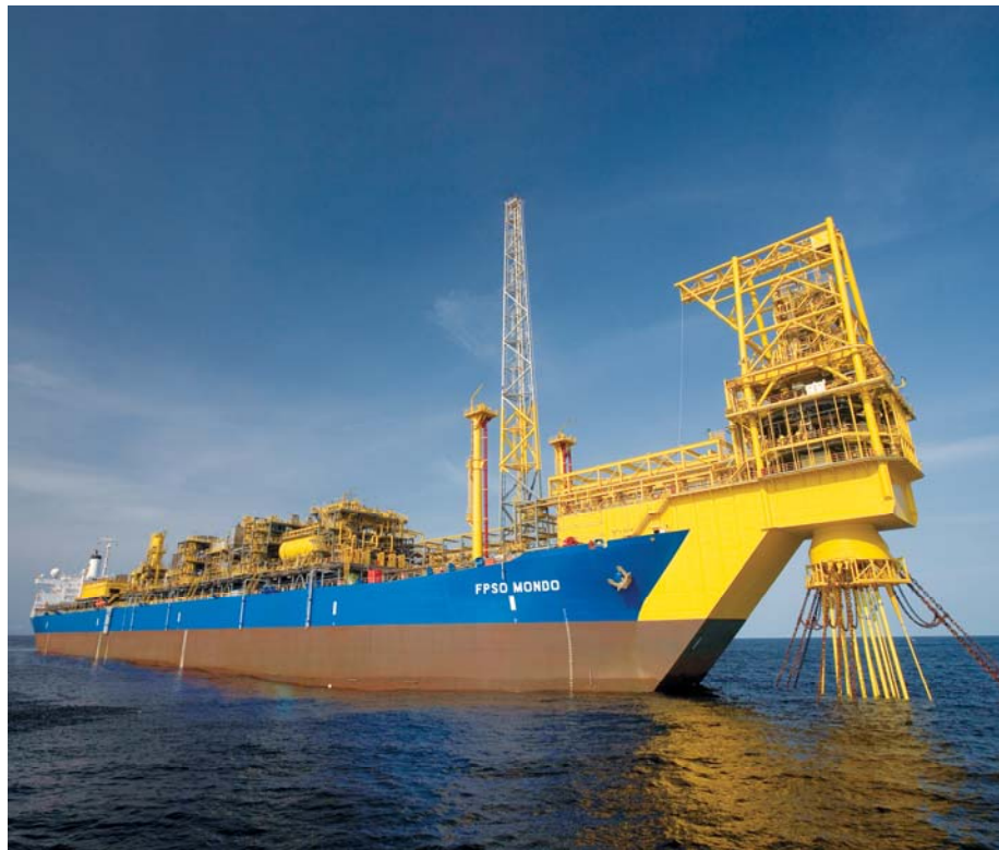
Mondo FPSO vessel at Kizomba Satellites Phase 2, Angola
