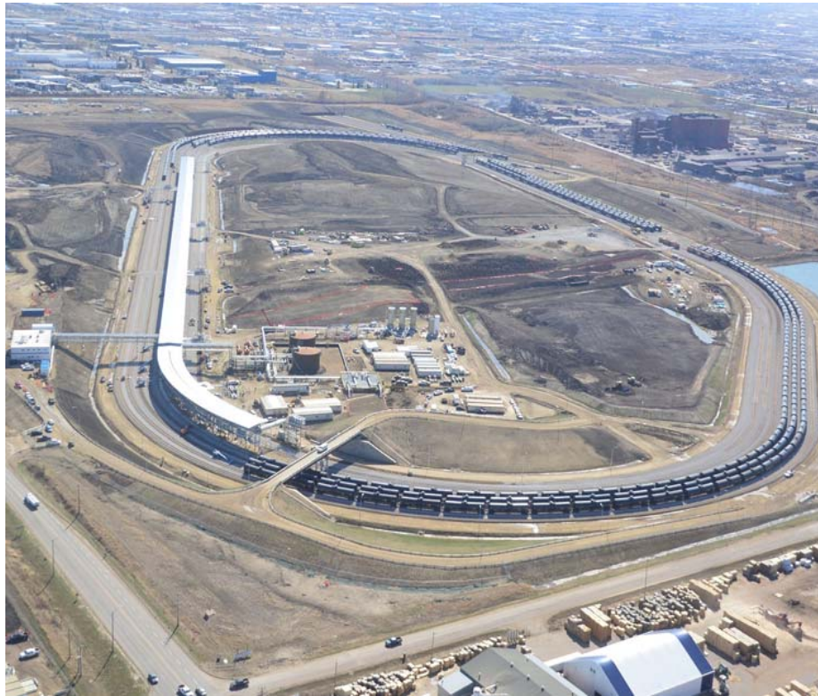
Edmonton Rail Terminal, Canada
